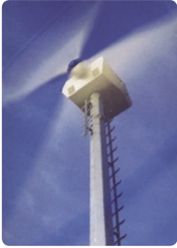
Wind turbine with galvanised steel ladder
